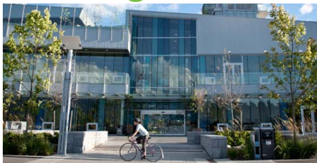
Creekside – 2010 – LEED Platinum
