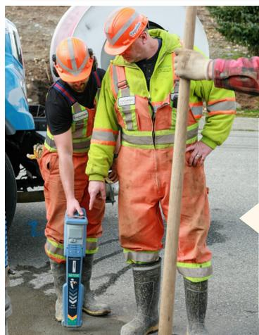
Crews are trained to use specialized tools, such as this radio detection device, to locate underground utilities. By using these tools, the crew can better detect the location of utilities, to avoid unnecessary outages for the community.
