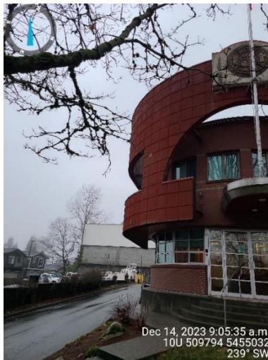
Photo 1: Austin Heights Fire Hall Facade
