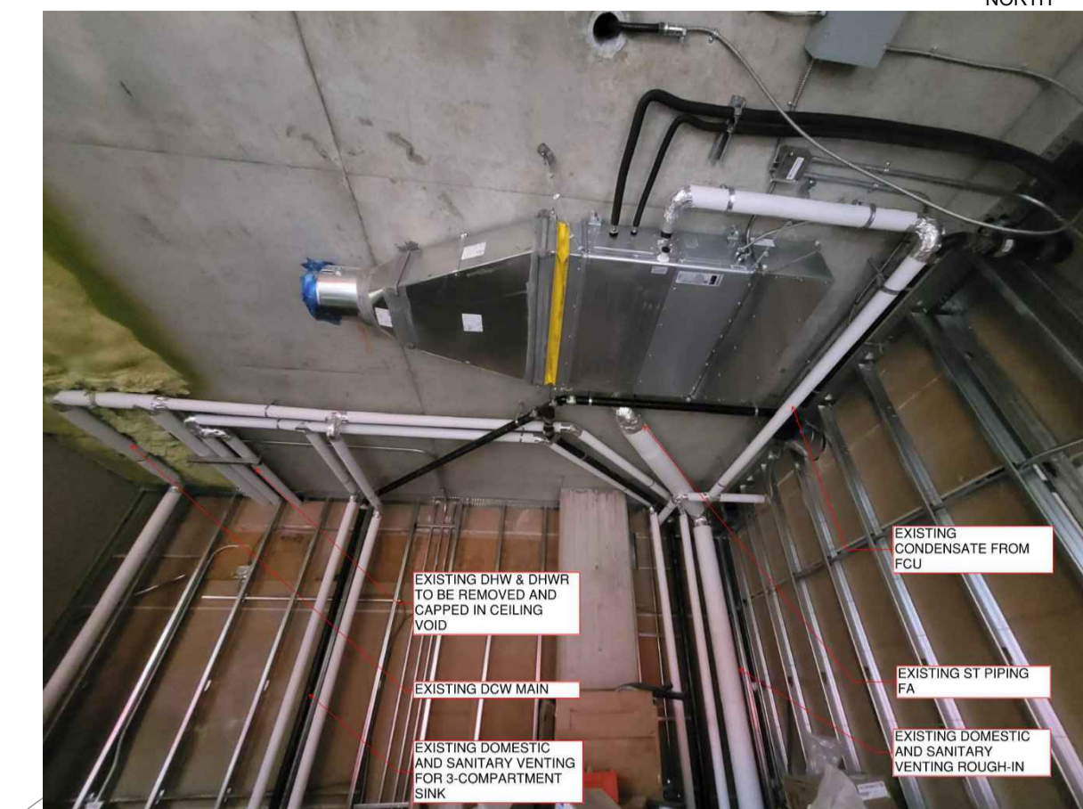
EXISTING PLUMBING - CONCESSION STAND - LEVEL 1 M101 SCALE: NTS
