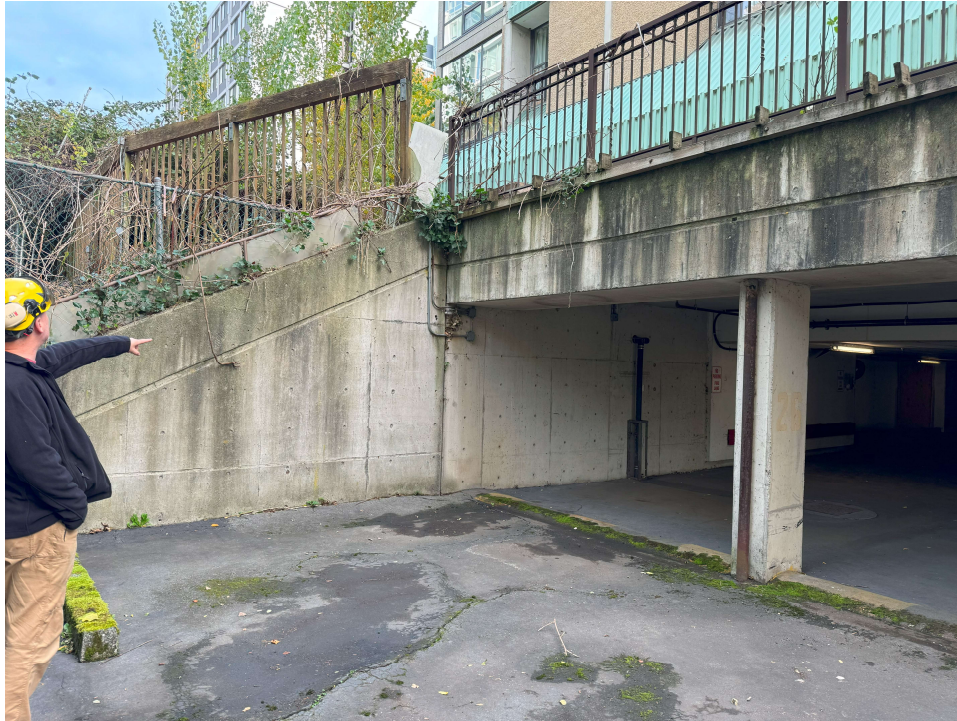
Photo 3 View north, showing northern “wing wall”.
