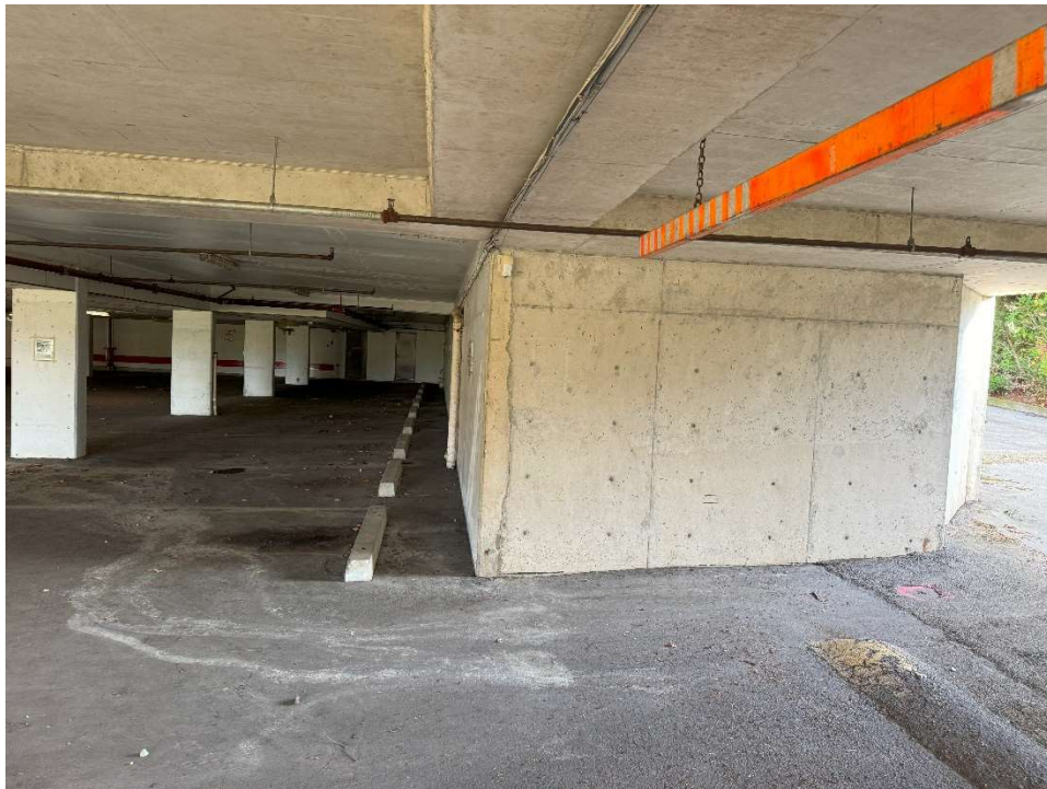
Photo 2 View north, showing basement walls.
