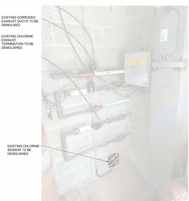
**EXISTING CHLORINE SENSOR** M101 SCALE: NTS
