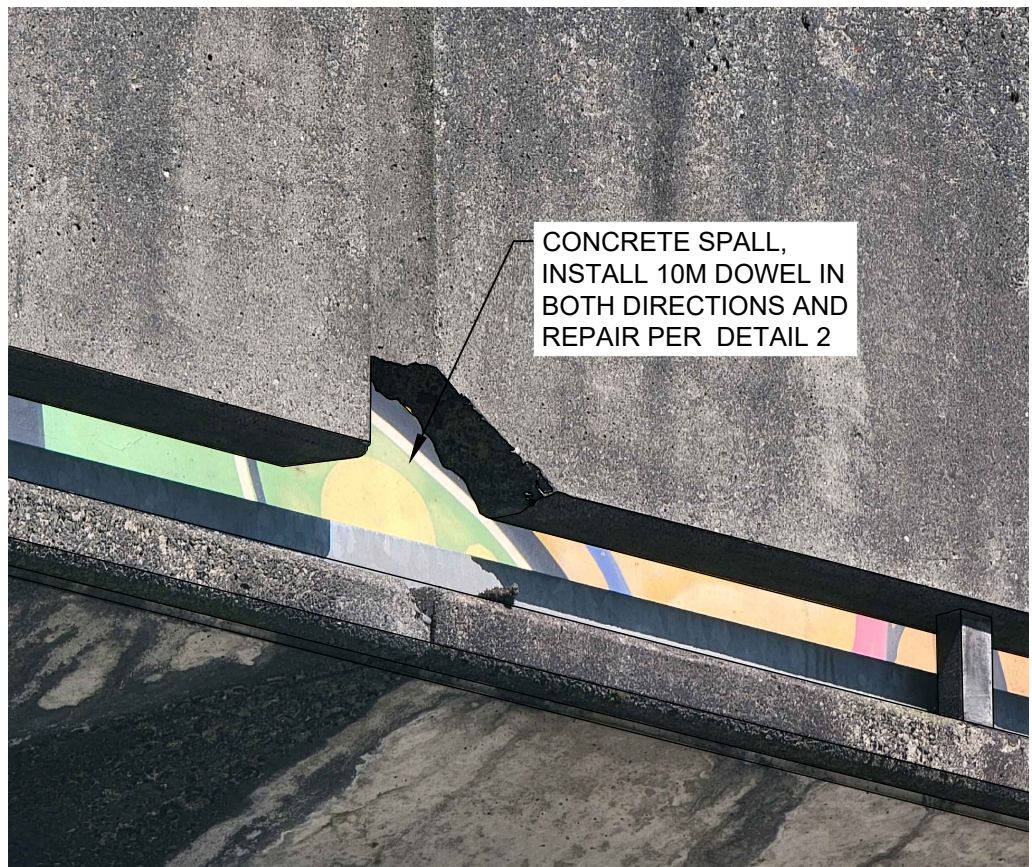
PHOTO N.T.S. HORIZONTAL CONCRETE SPALLING AT PARAPET, TYP
