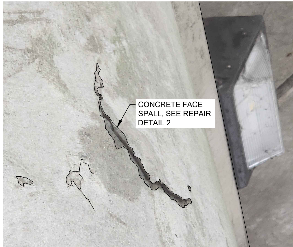
PHOTO N.T.S. VERTICAL CONCRETE SPALLING AT FACE OF PIER, TYP
