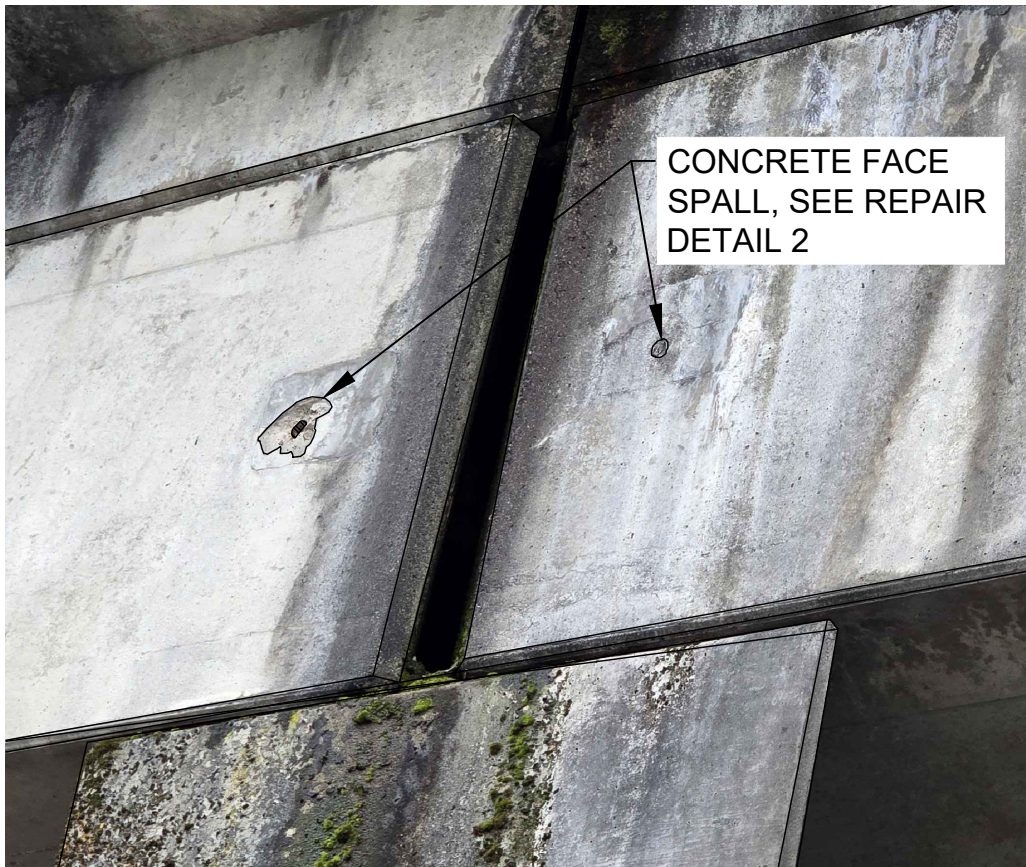
PHOTO N.T.S. VERTICAL CONCRETE SPALLING AT EXTERIOR FACE OF GIRDER, TYP
