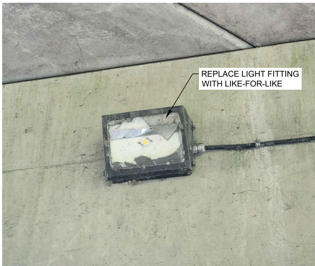
PHOTO N.T.S. REPAIR EXISTING LIGHT FIXTURES
