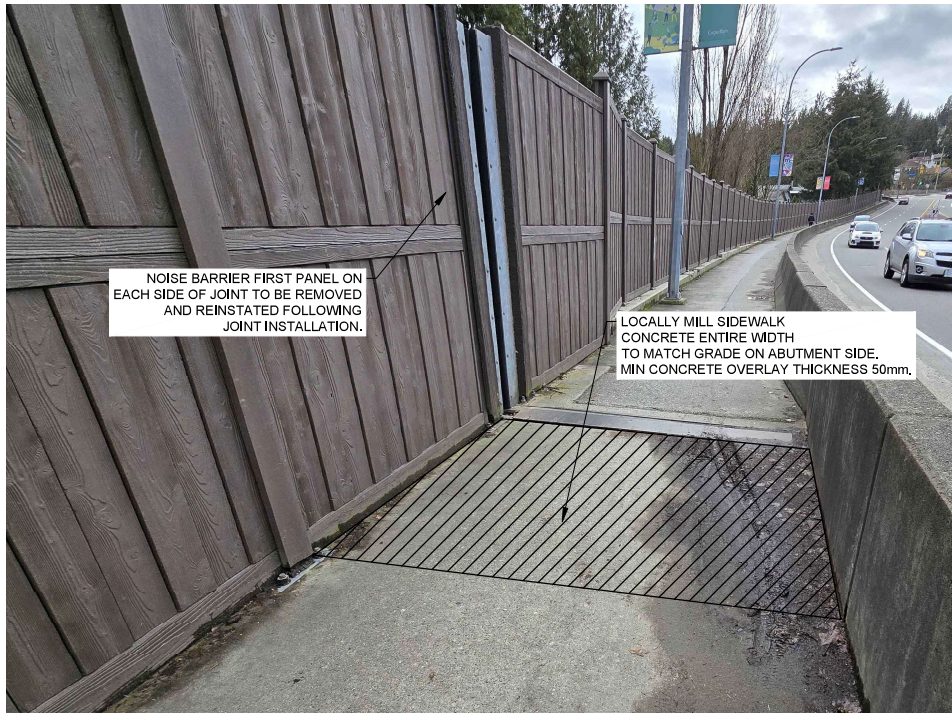
SIDEWALK CONCRETE OVERLAY EXPANSION JOINT AT SOUTH ABUTMENT
