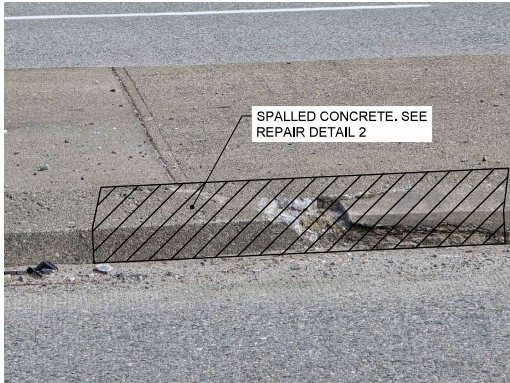
CONCRETE REPAIR NORTH END - MEDIAN
