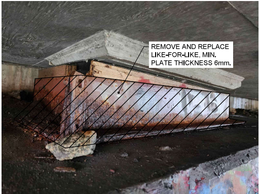
REPLACEMENT OF BEARING KEEPER PLATES NORTH ABUTMENT
