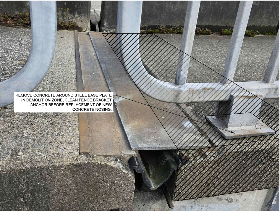
STEEL FENCE ON SIDEWALK EXPANSION JOINT AT SIDEWALK
