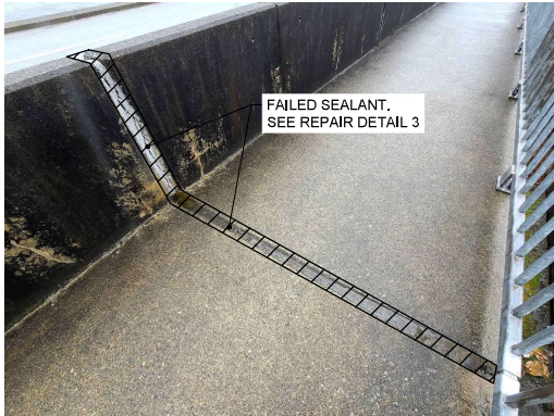
SEALANT REPLACEMENT PARAPET AND SIDEWALK
