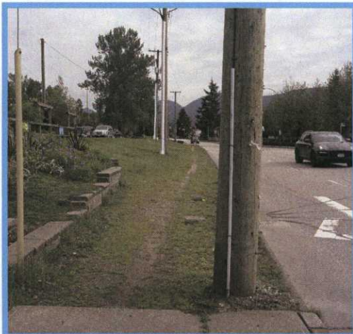
GAPS IN SIDEWALK
