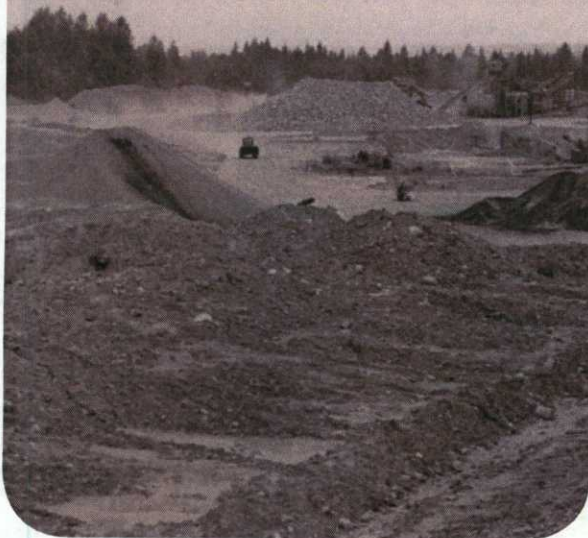
Lafarge Gravel Quarry Site
