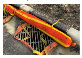
2. Sediment Barrier Berms/Check Dams – Berms or check dams in the context of inlet protection refer to the installation of temporary barriers installed in conjunction with filter sock inserts to augment the intended function of the inlet protection measures. Berms may consist of rock mulch, fiber rolls, or straw wattles installed along the rear openings of storm inlets to preclude the bypass of sediment laden runoff past filter sock inserts.
