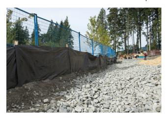
Critical to the function of silt fencing is the proper installation and "key in" of the lower flap of the geotextile fabric. The fabric flap must be oriented upslope and keyed in, backfilled, and compacted as per manufacturer's specifications to preclude potential bypass or undermining during runoff events.
