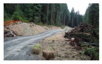
Interceptor ditches or swales must include design elements to minimize flow velocity or measures to mitigate channel invert and bank scour potential (see discussion re: Interceptor Ditches/Swales in section 4).
