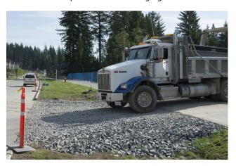
Rock mulch pads require frequent inspection and repair/ replacement to maintain their function and preclude offsite tracking.
