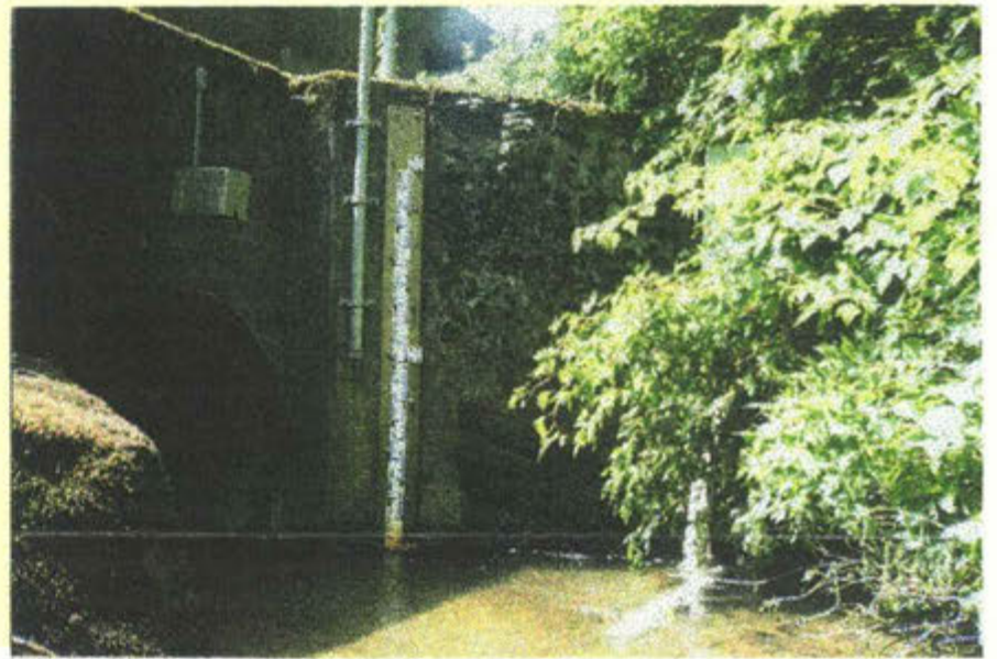
GVRD ULTRASONIC DEPTH GAUGE OVER WEST CULVERT
