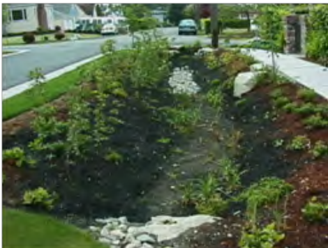
Flush curb (left) to grass filter to vegetated swale.
