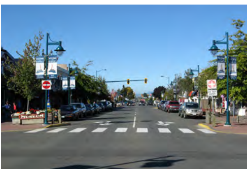
Asphalt Driving Surface
