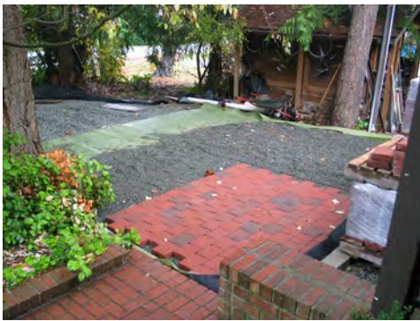
Pervious paver installation
