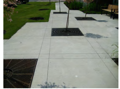
Scored concrete can be used to define areas or create a specialty paving look.
