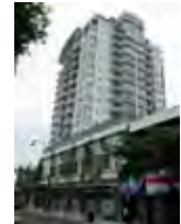
The tower and podium form accommodates a large number of homes above shops and offices. This supports convenient transit service to and from the neighbourhood centre.
