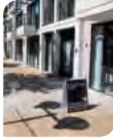
The main floor of a ground-oriented unit can be used for either work space or extra living space and provides an incubator space for small, local business. When designed properly a live-work unit can look like a regular townhouse.
