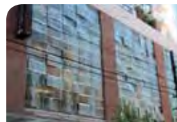
The art glass wall on this building screens an above grade parking garage.
