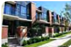
These ground-floor patios allow for personalized landscaping and help to lend a residential character to the street and increase the feeling of safety in the neighbourhood.
