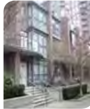
Having the main floor of a ground-level unit raised up can help to increase privacy and the separation between public and private space.
