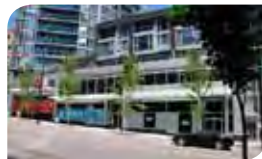
The building slab steps down allowing each shop to meet the grade of the sidewalk.
