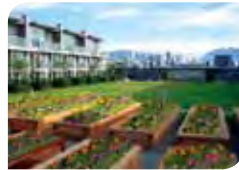
A large roof with natural landscaping helps to cool the building in summer and providing extra insulation in winter while giving residents gardening plots and recreation space.
