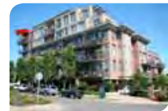
The top of this building steps back to reduce shadowing and the perceived size of the building at street level.
