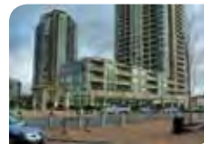
The placement of these towers on opposite corners of the podium helps to minimise shadows and ensure a degree of privacy for residents.
