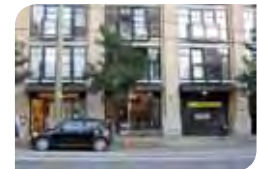
This garage entrance is small and matches the pattern of the rest of the building while respecting the adjacent retail shops.
