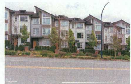
3.2.3 b Buildings are stepped on sloping sites to reduce height and massing
