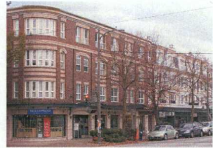
Demonstrates a strong consistent streetwall across multiple buildings
