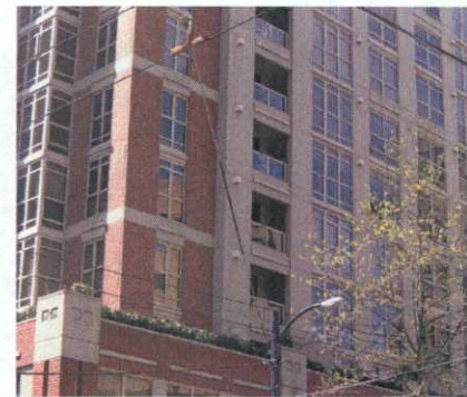
Demonstrates inset balconies
