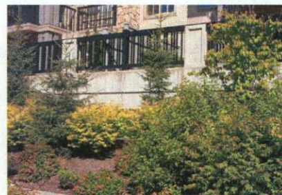
4.3.1 d Exposed Foundation Walls
