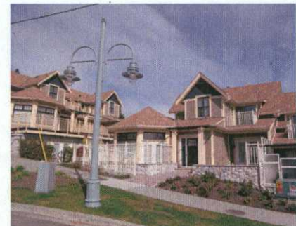
Demonstrates a steep pitched gable roof and traditional styled wood siding with heavy trim
