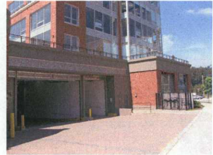
2.7.2 a Loading and service areas located at the rear of the building
