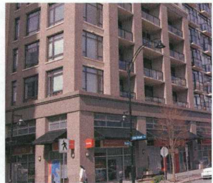
Demonstrates inset windows with dark frames that are oriented vertically grouped into a consistent rhythm
