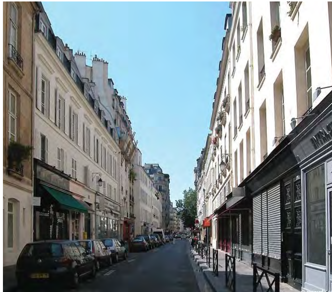
Continuous street wall
