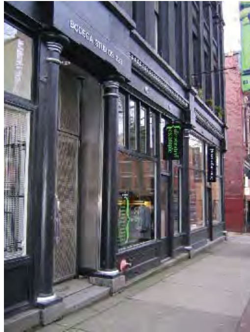
Steel beams over retail openings and structural columns are expressed
