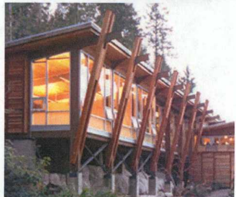
Demonstrates wood soffits and exposed structural supports
