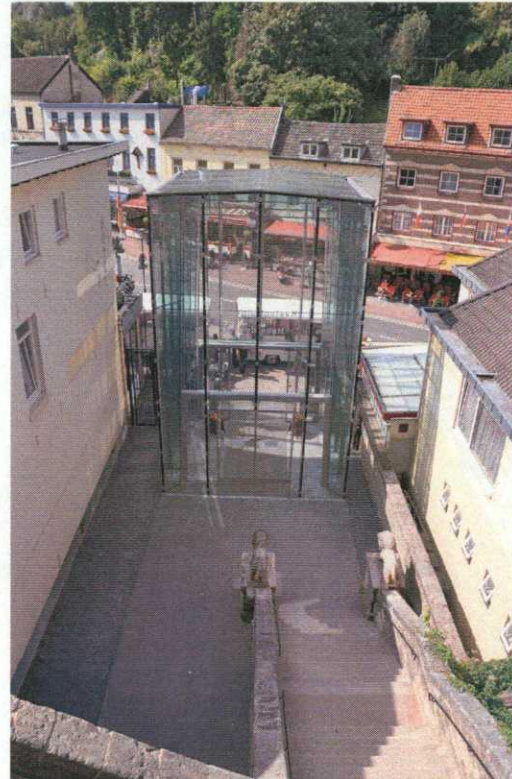
Example of a public elevator in a hillside commercial centre (Illustrative concept only)
