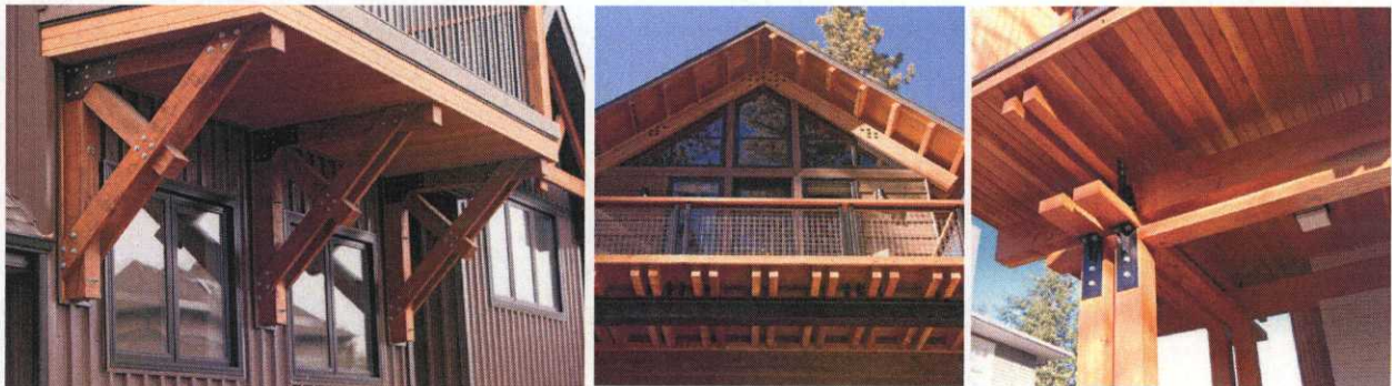
Illustrates wood roof and balcony soffits
