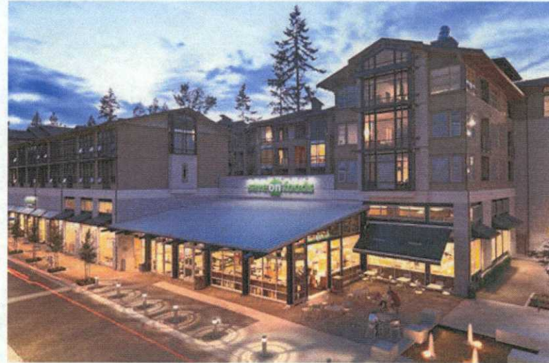
Precedent for a grocery store that engages an outdoor plaza with a high degree of transparency (Illustrative concept only)
