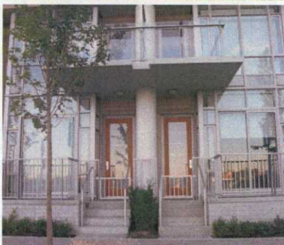
Demonstrates treatment of ground level units
