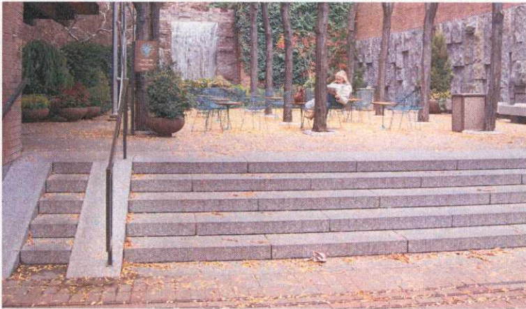
Demonstrates bike channels for ease of movement up and down stairs
