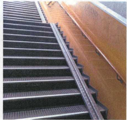
Demonstrates bike channels for ease of movement up and down stairs
