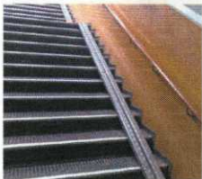
Examples of bike channels for ease of movement
