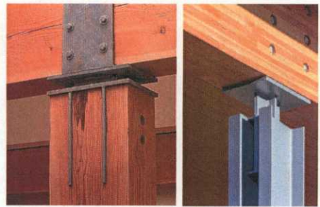
Demonstrates well crafted timber details
